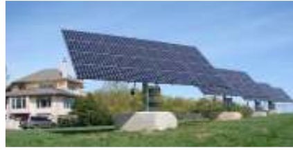
Gambar 3. Solar Tracker Dua Axis
